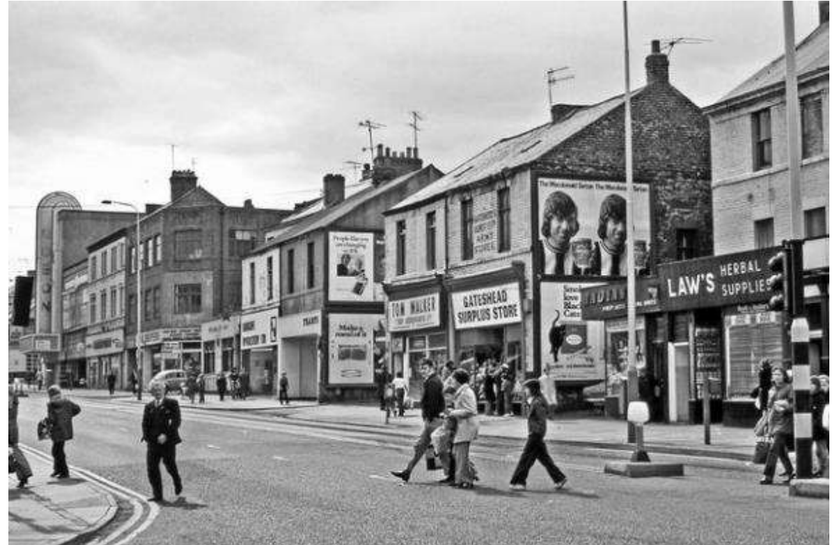
West side of HSS looking south c1960
